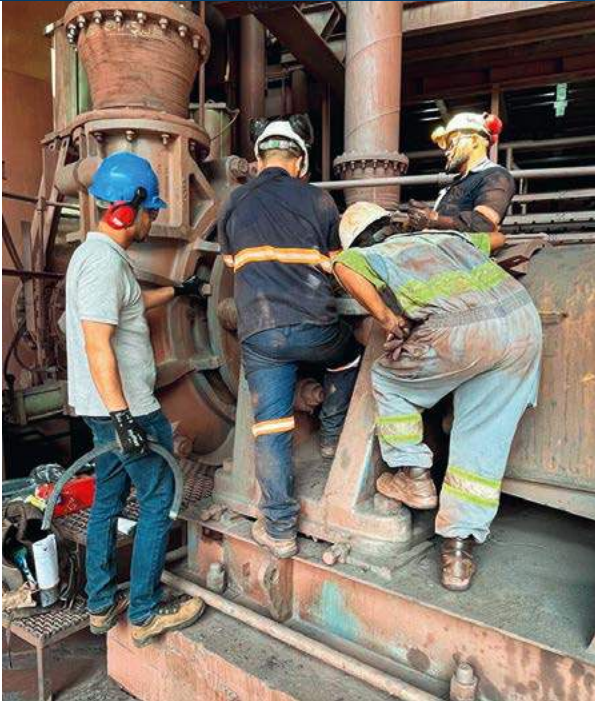
Vinicius Tomiati (left) oversaw the installation of the packings at Vale's Cauê Mine in Itabira, Brazil.
