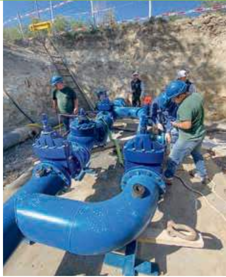
The DN 300mm pressure reducing station will connect the main reserve to a secondary reserve in Puerto Madryn.
